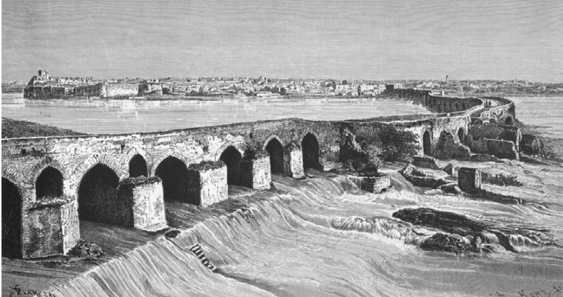
Figure 5. Bridge-dam of Shâdorvân in 1880s, (Dieu la Foie and from the nomination file, SP of Iran)
