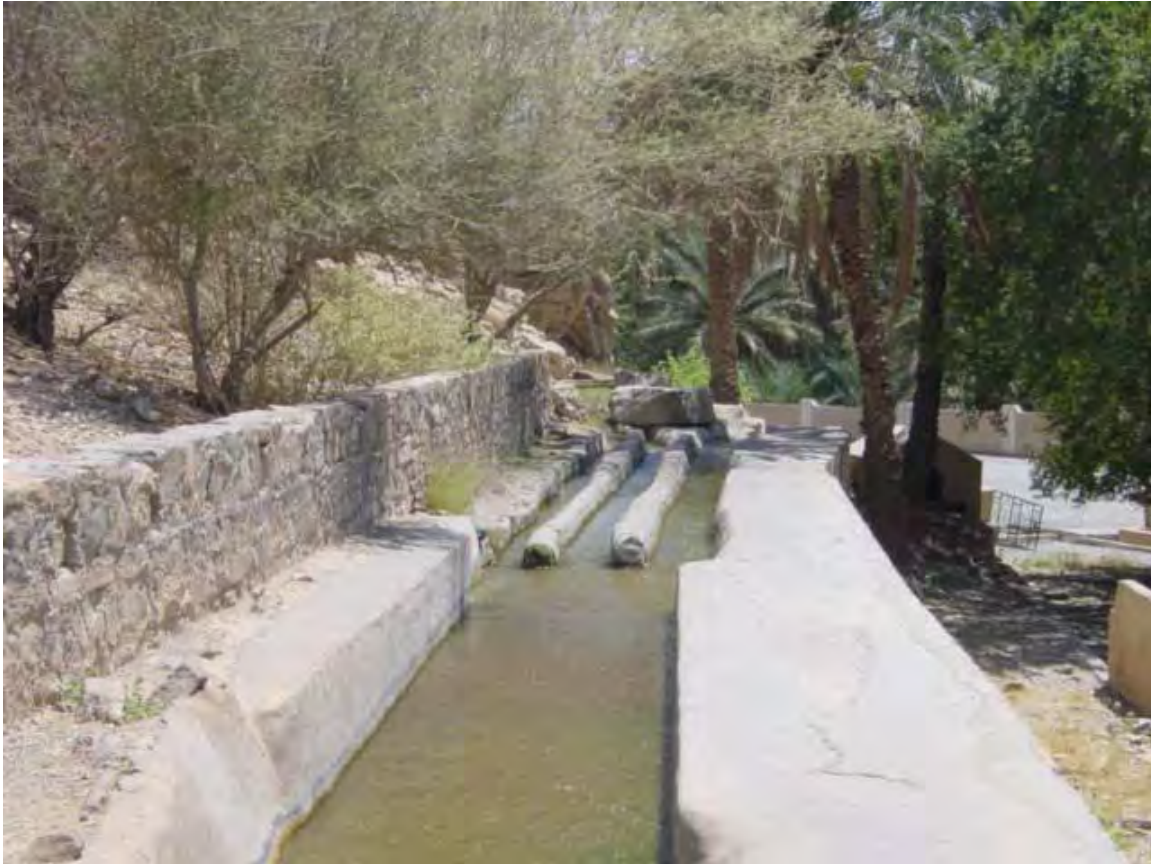
Figure 4. Falaj Al-Khatmeen, distribution point at the end of the shari'a (nomination file, SP of Oman)
