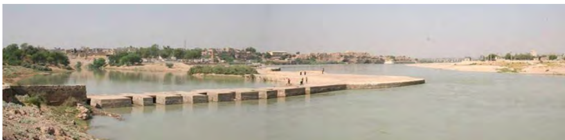
Figure 4. Mizân water intake dam at the entrance of the artificial Gargar River (nomination file, SP of Iran, ICHHTO)
