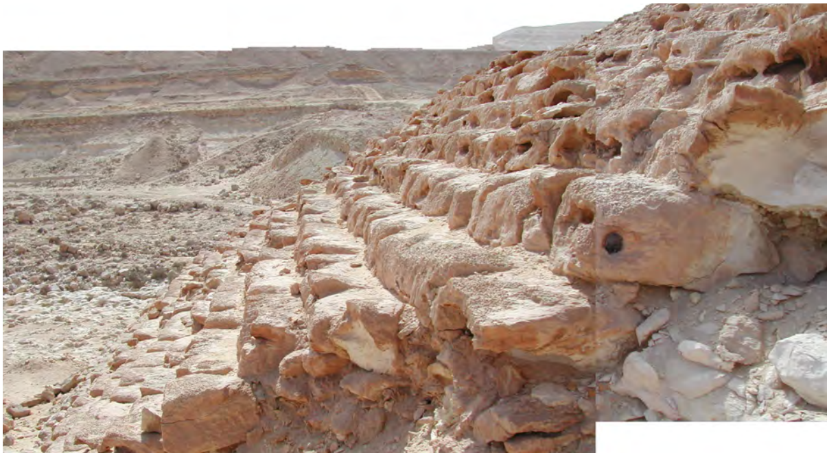
Figure 1. Wadi Garawi (Sad el-Kafara ) Dam, Helwan, South of Cairo (Fekri
