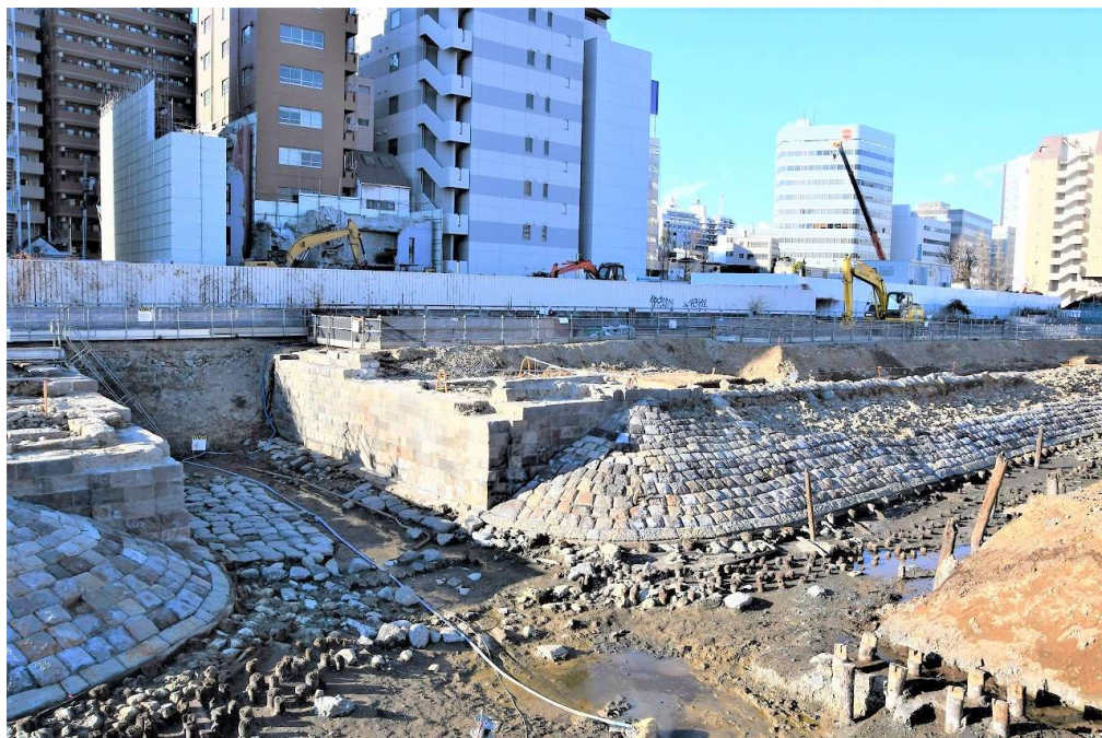
Bridge section in Block 3 (from east), to be partly preserved
